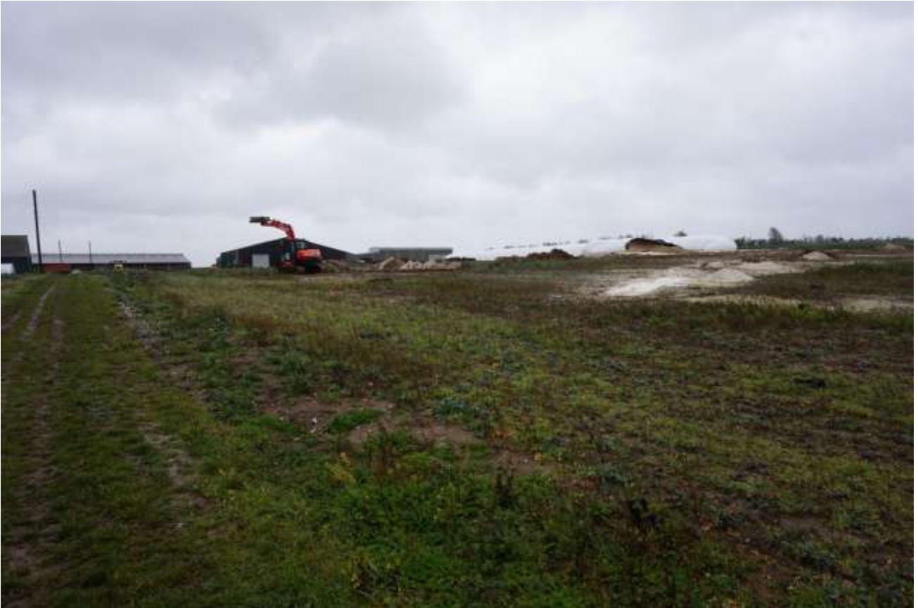
Plate 1: Looking north east at the site from its southern end
