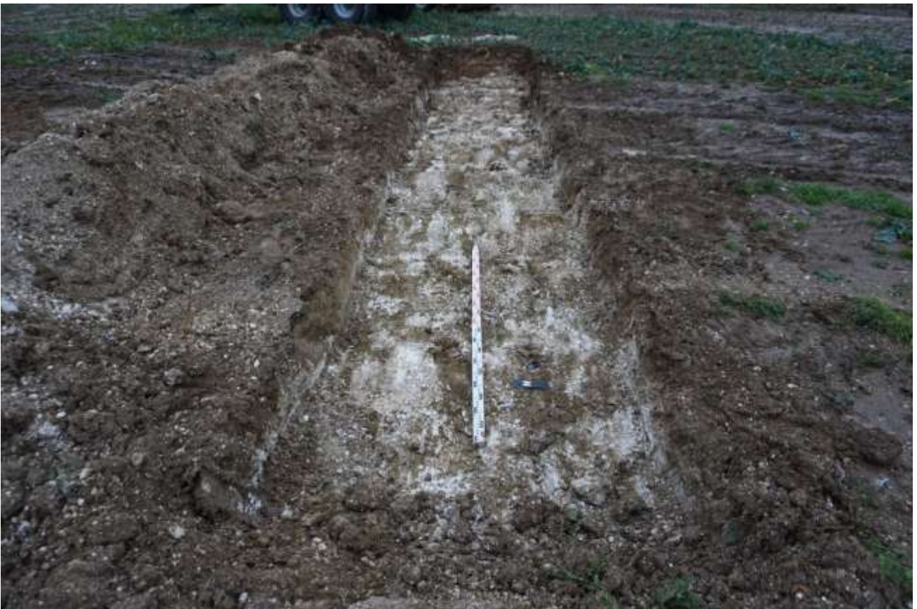
Plate 4: Looking east at trench 2
